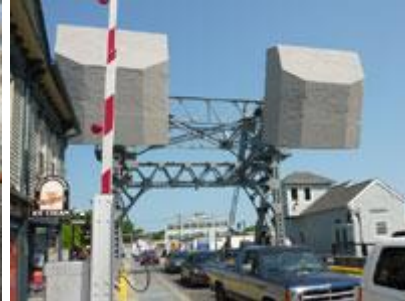
Lift bridge at Mystic
